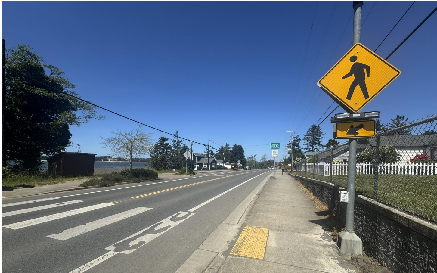
Post Mount Rapid Flashing Beacon (RRFB)
